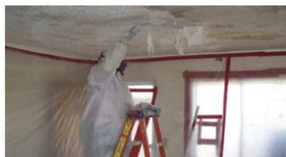
A P.W. Stephens Environmental technician removes asbestos from a client's ceiling.
