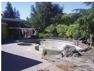
Dig & Demo recently worked on this pool demolition/removal project.
