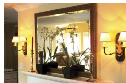
All In One Home Services installed these two outside sconces in a client's home.
