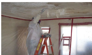
A P.W. Stephens Environmental technician removes asbestos from a client's ceiling.
