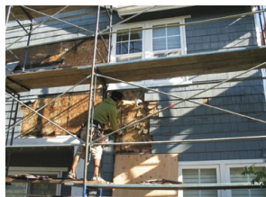
A tear down and new exterior project by IRC All Siding
