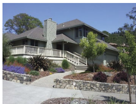
A recent exterior painting project by E.G.I Custom Painting
