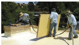
Abрил Roofing's technicians install a polyurethane foam roof.
