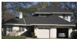
Northern California Roofing recently installed this roof on a client's home.
