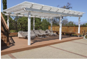
A recent deck and arbor project by M&M Builders
