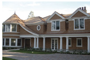
A recent wood shingle and siding project by Mid-Peninsula Roofing
