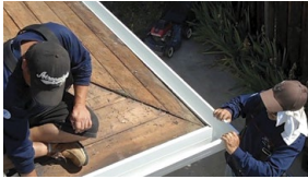
Two Gutter Pros technicians work on a client's gutter project.
