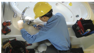
Drain Doctor's technicians can perform all types of plumbing repairs.
