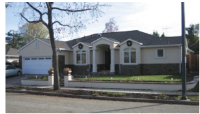
A recent residential remodeling project by An Ky Construction
