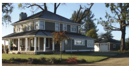
Penny Pinching Construction & Remodeling recently completed work on this house and garage project.
