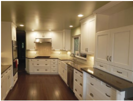
MDS Construction recently completed this kitchen remodeling project.
